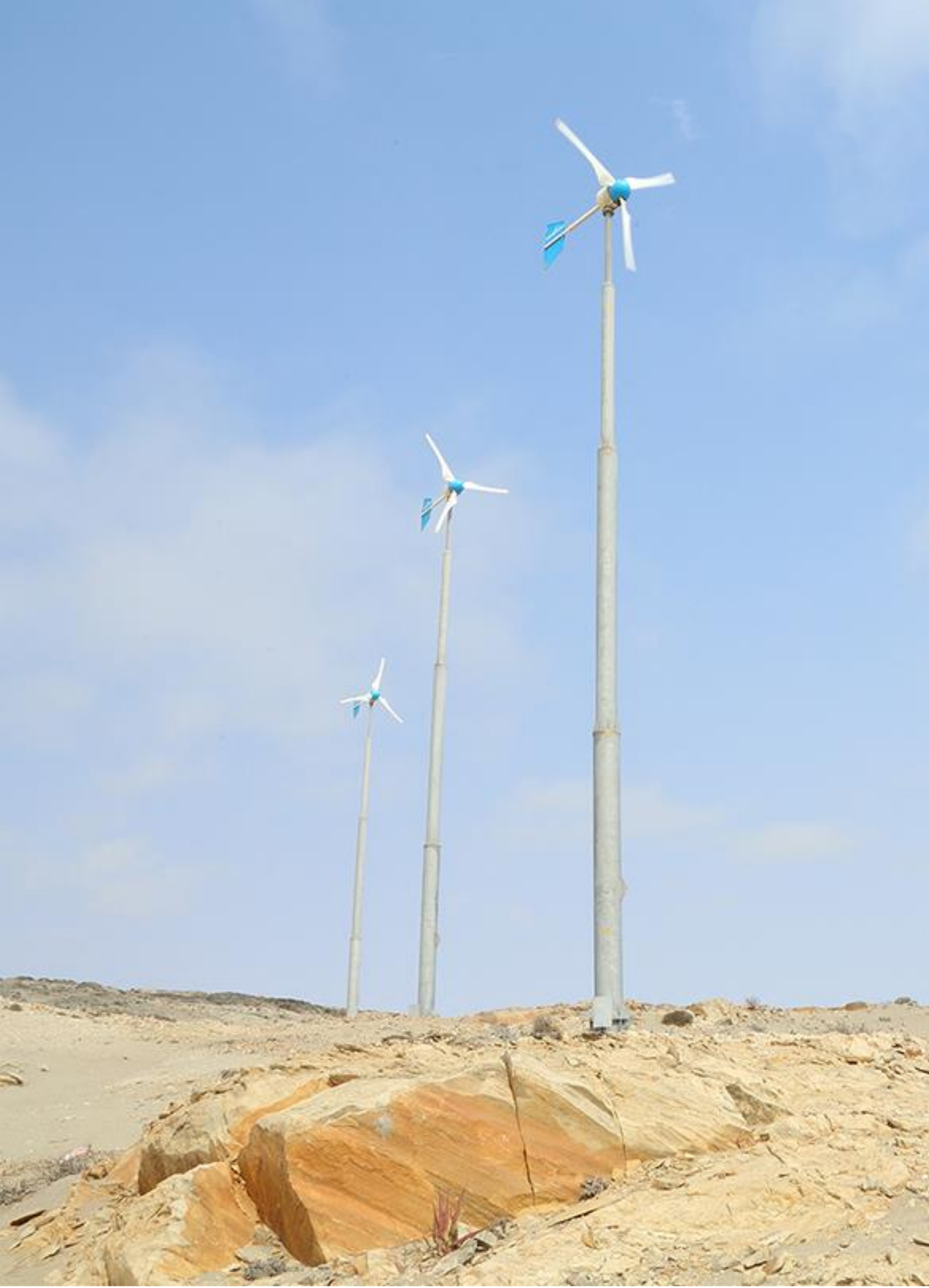
3.5 kW per turbine, total rated power = 10.5 kW. 5 community technicians trained on operation & maintenance of the wind power plant
